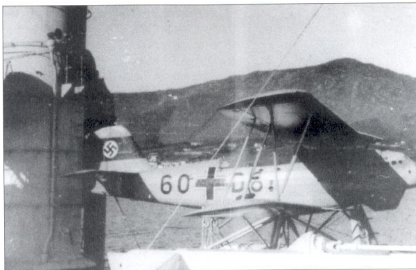
A close-up of Leipzig 's Heinkel He 60 floatplane sitting in its launch cradle on the catapult, just ahead of the funnel. The aircraft is in its pre-war pale grey livery. The biplane He 60 was later replaced by the far superior Arado Ar 196.
